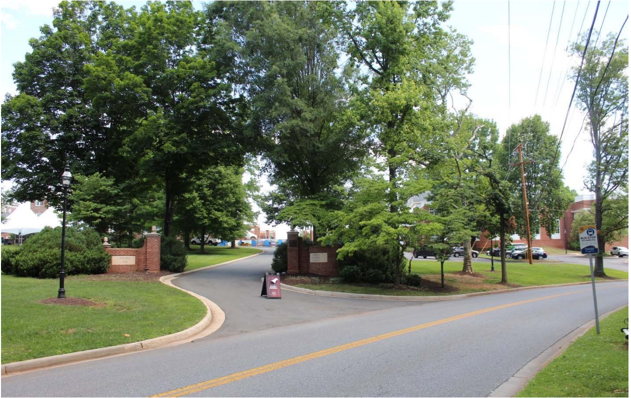
Figure 5-96: Photo location 1- View of VES campus entrance, facing north.
