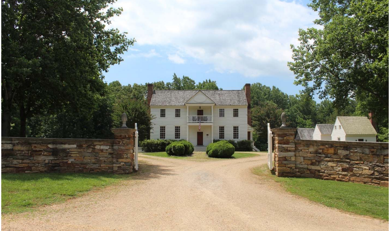
Figure 5-77: Photo location 1- Bowling Eldridge House, front façade, facing south.
