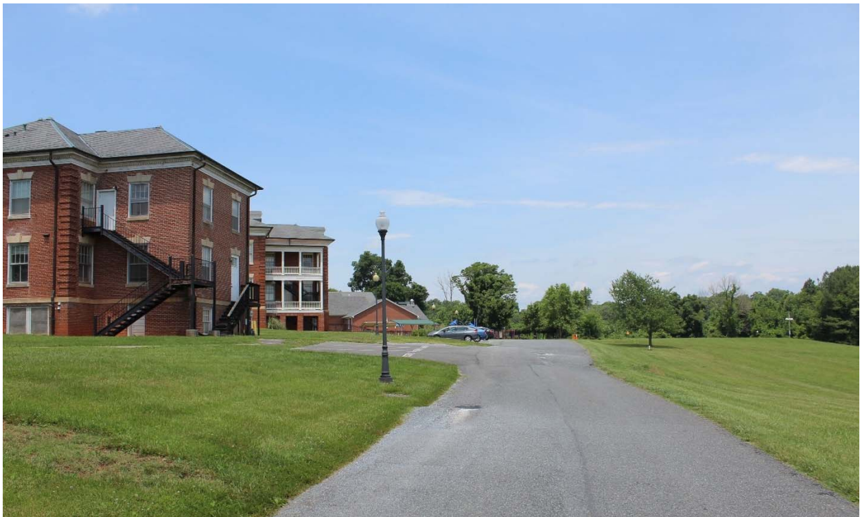
Figure 5-115: Photo location 4- View from rear driveway towards the Project (not visible – screened by vegetation), facing north.
