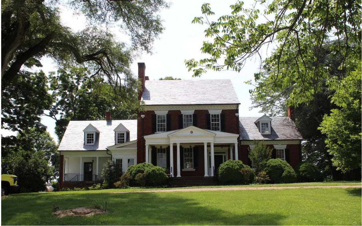
Figure 5-2: Photo location 1- View of Elk Hill, front façade, facing west.
