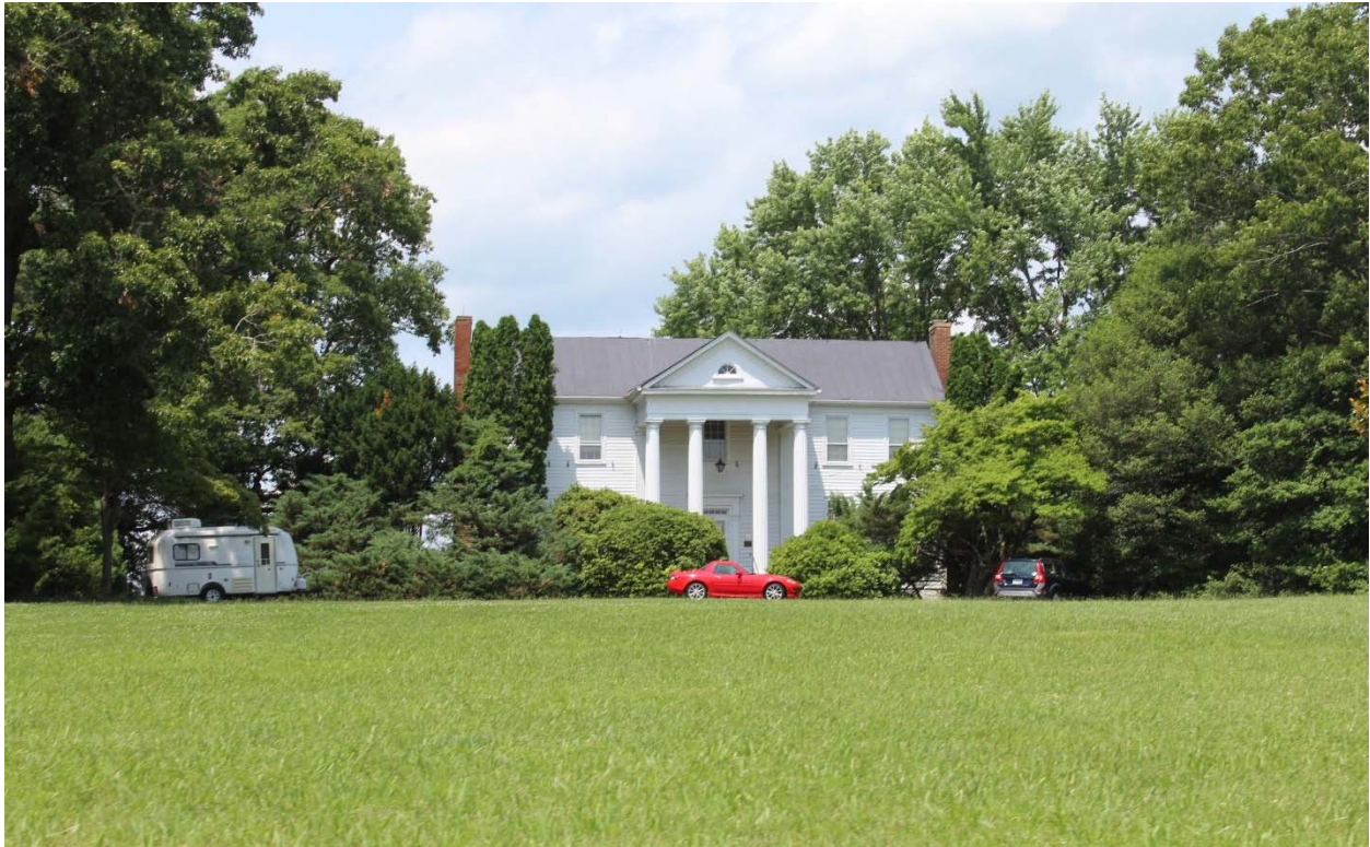
Figure 5-44: Photo location 1- View of Old Rectory, front façade, facing north.
